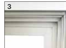
3 Check Angle for 90 degrees
