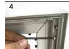
4 Fit off with allen head screw
